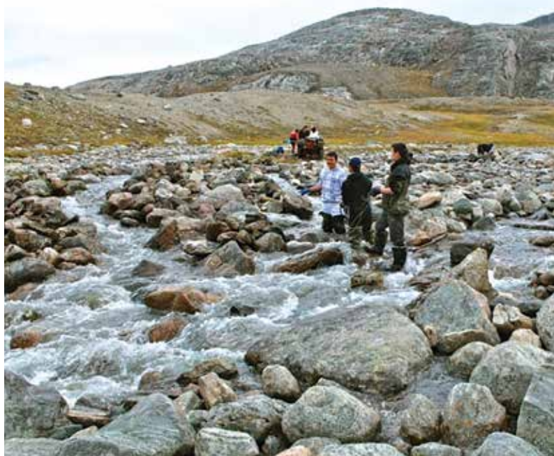
A channel was dug manually by youth in a creek near Kangiqsujaq in 2012.
